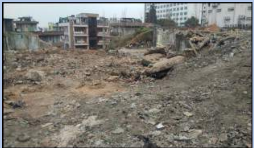
Site Clearance Works at MTC Land
